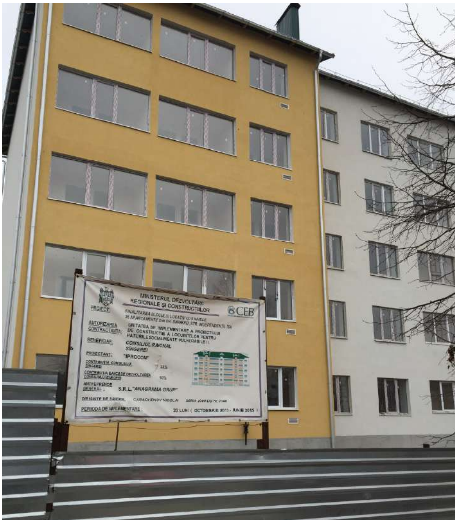
Picture 1. A housing construction project for socially vulnerable segments of the population
